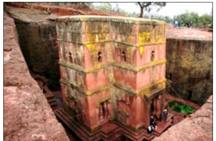
9.114 St George's church in Lalibela (Ethiopia) is a rock-hewn building, creating by excavation from the surrounding stone.
