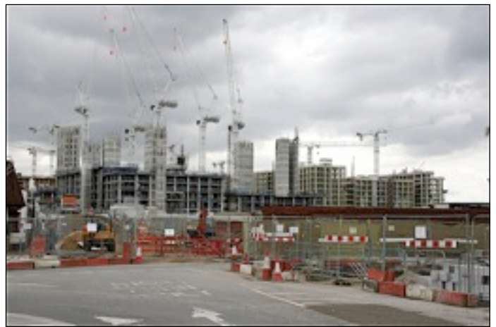
9.26 The Athlete's Village, under construction for the London Olympic Games of 2012.
