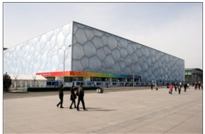
9.24 The National Aquatic Centre, also known as the Water Cube, is an example of urban infrastructure from the 2008 Olympics in Beijing.
