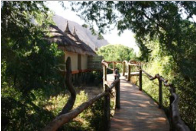
9.55 These cabins at Serra Cafema have been built on stilts above the banks of the Kunene River (on the border of Angola and Namibia) to protect the riverbank ecology and avoid problems from floodwaters.
