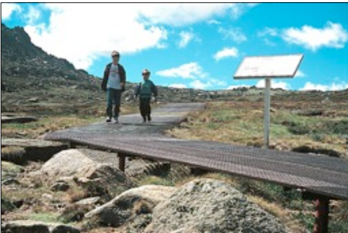
9.79 An elevated pathway has been built to protect the fragile alpine ecosystem of Mount Kosciuszko (Australia) from damage by tourists.
